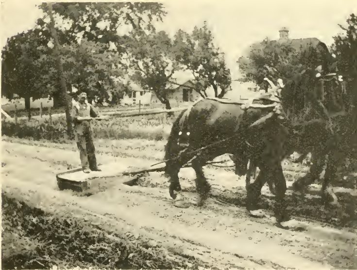
Fig. 40. King Road Drag in Use.
